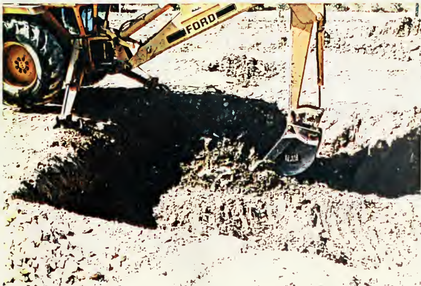
A2: COVER EXCAVATED TO GARBAGE LAYER
